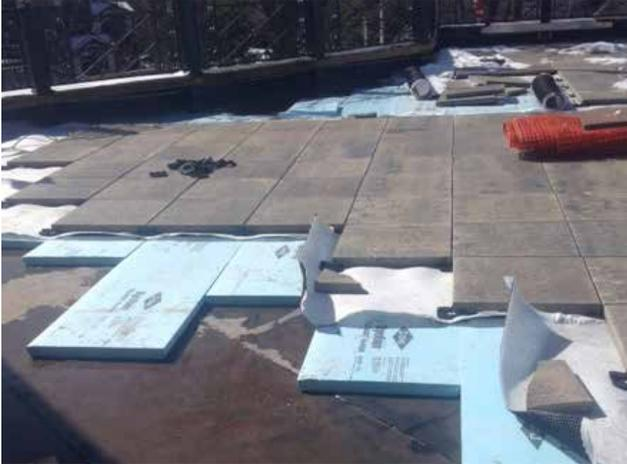
*PTO Roof System installs over existing roof*
