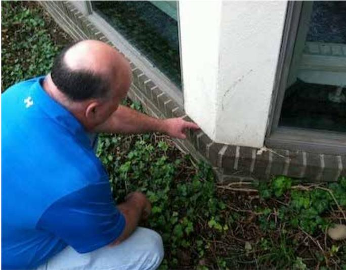
*Pointing out moisture infiltration at brick and EIFS interface*
