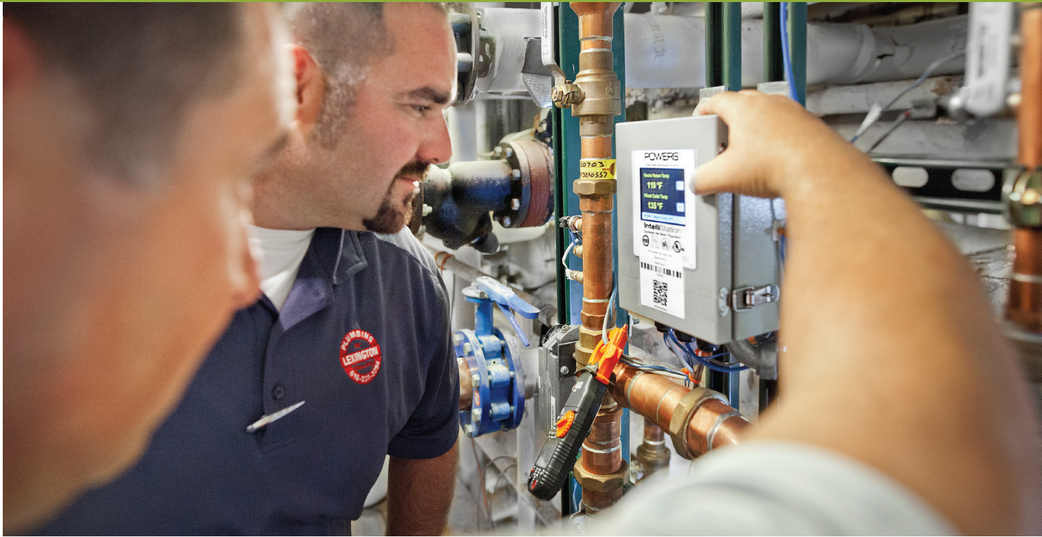
After making adjustments to the mixing valve, Ian Walters, project manager, Lexington Plumbing (center) and Jamey Shibel, outside sales for the manufacturer's rep firm, Mack McClain and Associates, determine the domestic water temperature setpoint.
