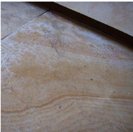
It is a common condition on new stone installations or when the stone has been exposed to a large amount of water, such as from flooding. This powder is actually a mineral salt from the setting bed.
