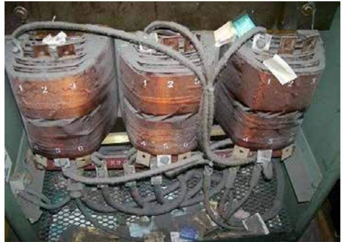
*Dust and Dirt Can Accumulate Causing A Potential Fire Hazard*
