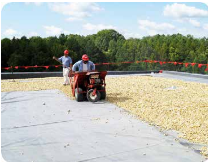
Loose-laid stones ballast EPDM roof system
