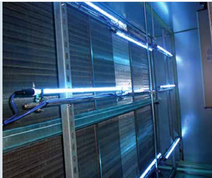
UVGI is effective for microbial disinfection of interior wall surfaces, coils and the supply airstream of air handlers
