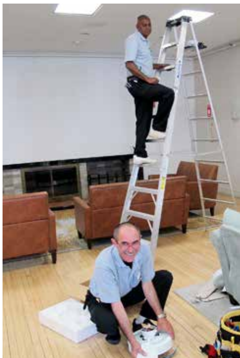
Ramon and Nikolay installing a ceiling fan
