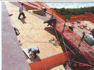
Installing new decking
