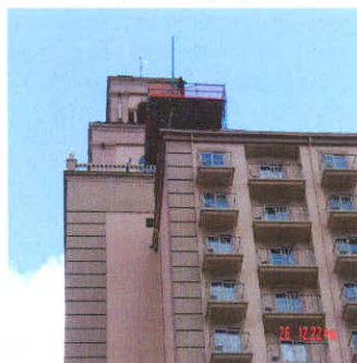
Roof top hydraulic hoisting stage area.
