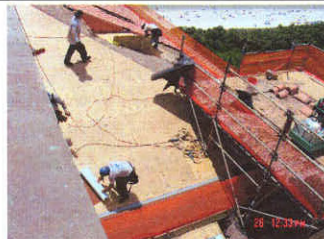
Installing new decking
