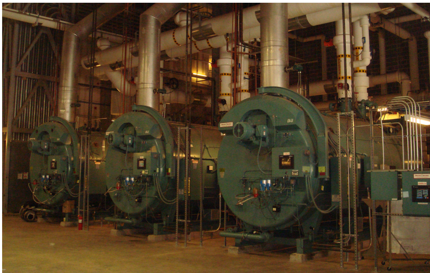
Gaylord's Heating Water Boilers...three (3) of the plant's six (6) total boilers
