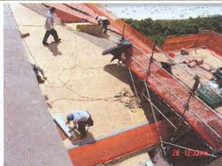
Installing new decking
