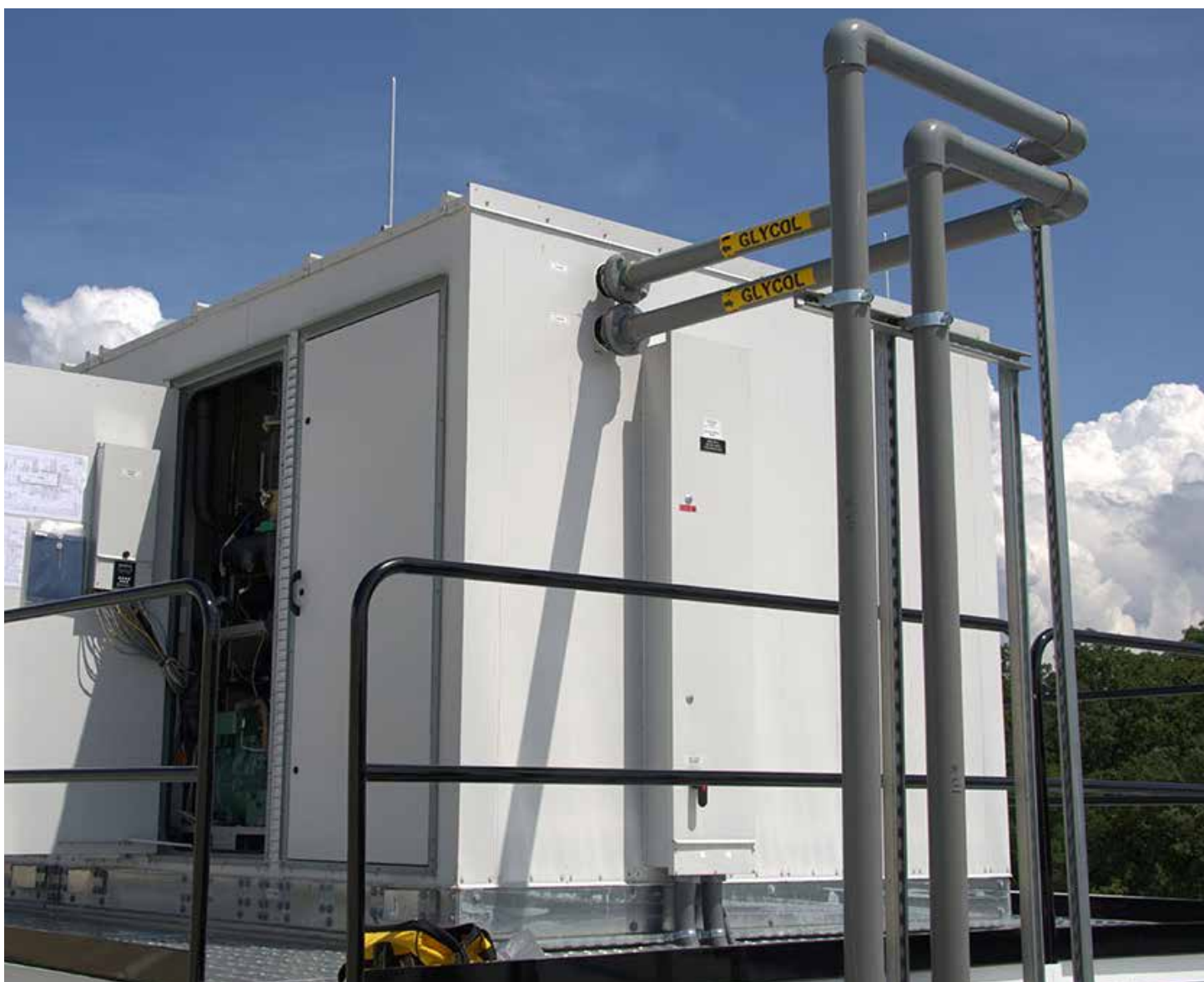
This rooftop dehumidifier system uses up to 85 percent less refrigerant by relying on glycol.
