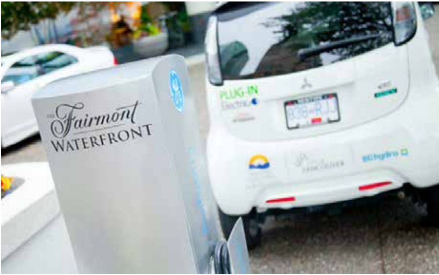
“Fairmont Hotel Electric Vehicle Charging Station”
