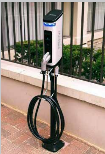
The standard J1772 receptacle can receive charge from Level 1 or Level 2 equipment.
