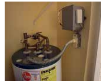
In addition to significantly reducing HVAC costs, GEM Link® also wirelessly controls the 3 kW electric water heaters at the Tropic Sun Towers.
